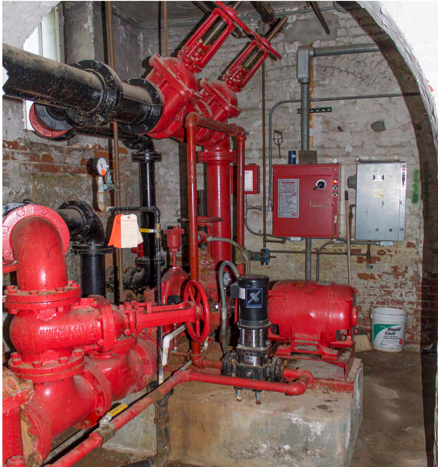
FIRE PUMP IN BASEMENT OF #14
