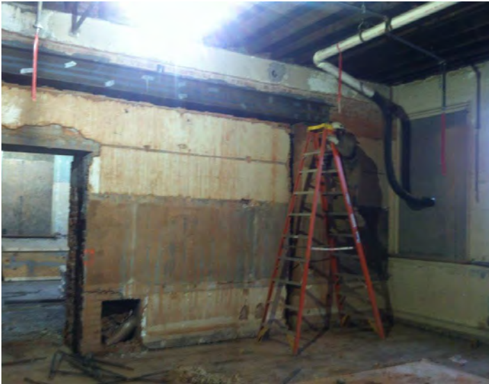
CONSTRUCTION PHOTO SHOWING REMOVAL OF BEARING WALL Walls were holding themselves up, but did not directly support floor loads.
