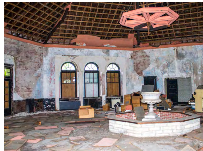
DAMAGE FROM MOISTURE INFILTRATION AT BUILDING #6
