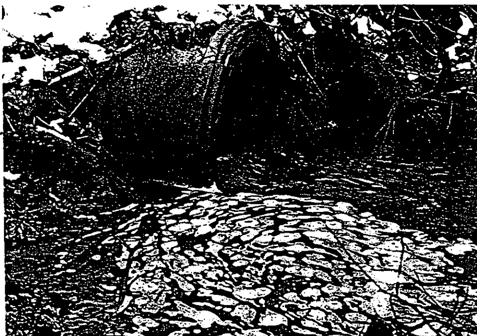
Orange foam forms around a drainage pipe that has to be regularly replaced because the water dissolves it.
