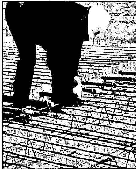
Dowel bar installation
