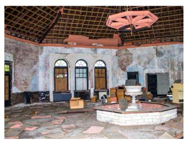
DAMAGE FROM MOISTURE INFILTRATION AT BUILDING #6
