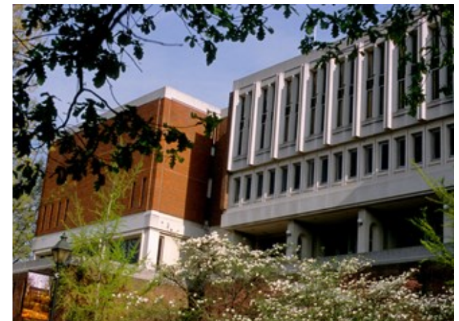
Above: Alden Library Phase 1.
