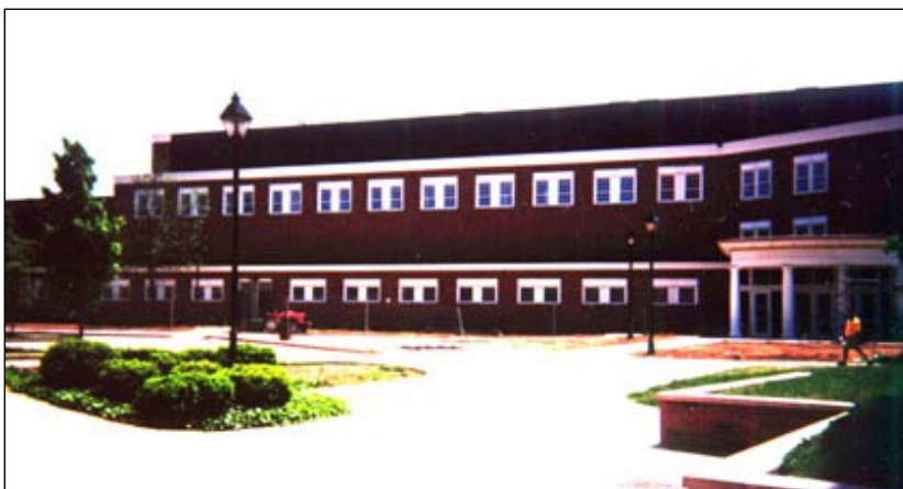
Grover Center is near completion as finishing touches are made to the outside of the building. Students and faculty can see the entrance facing Porter Hall.
