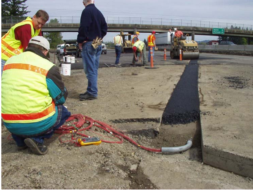
FIGURE 10 Trench and Conduit for the Strain Gage Lead Wires.
