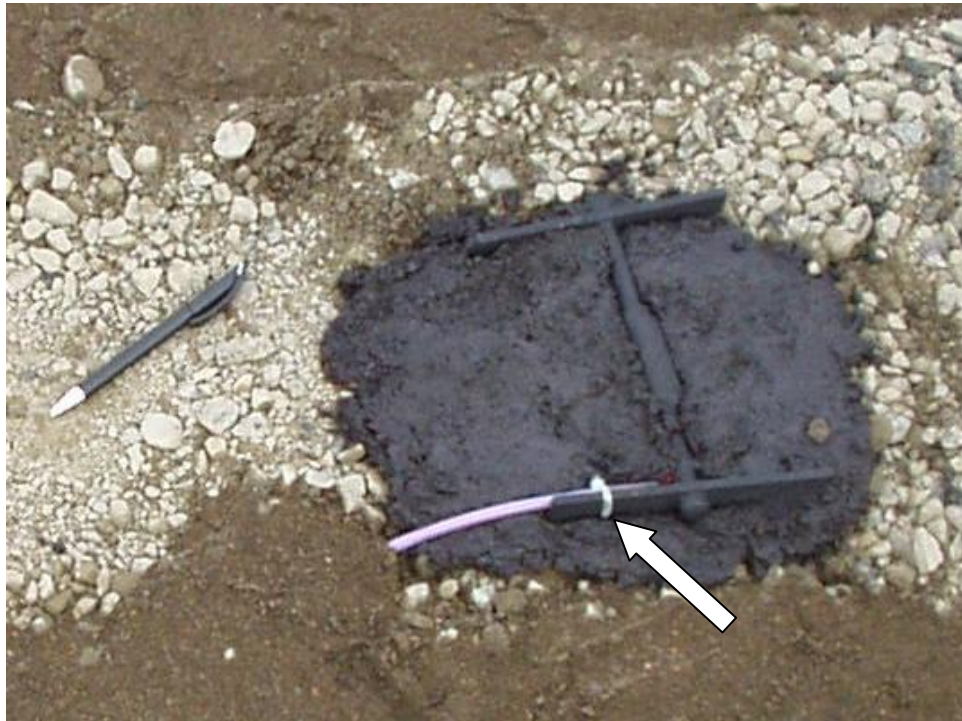
FIGURE 7 Sheathed Lead Wire Tied to the Strain Gage Bar.
