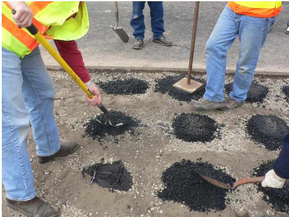
FIGURE 11 Initial HMA Placement and Compaction.
