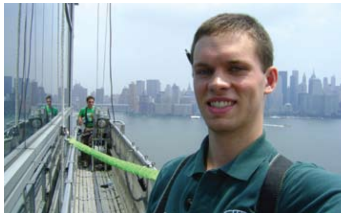
Top photo: Patrick Miner (left, white hat), checks work on the slurry wall at the Freedom Tower site in Manhattan.
