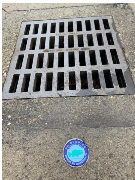
Figure 4: OHIO storm drain marked by an ambassador.
