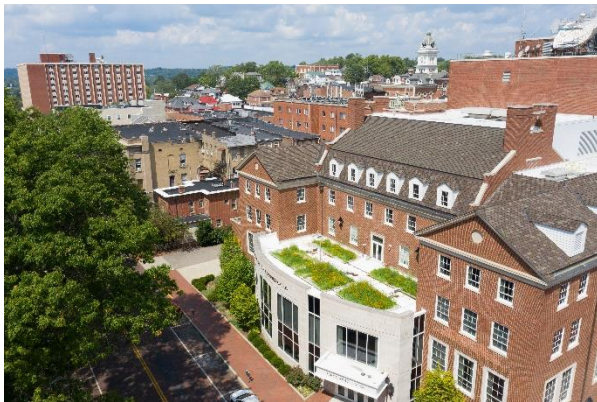
Figure 5: Schoonover Green Roof, 2020
